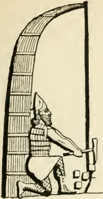
Soldier undermining a wall, sheltered by gerrhon .
